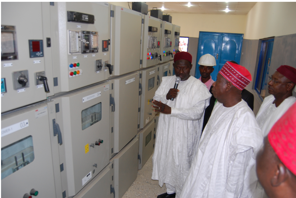
GOVERNOR GANDUJE LISTENING TO AN EXPLANATION DURING INSPECTION VISIT TO THE TAMBURAWA TREATMENT PLANT
