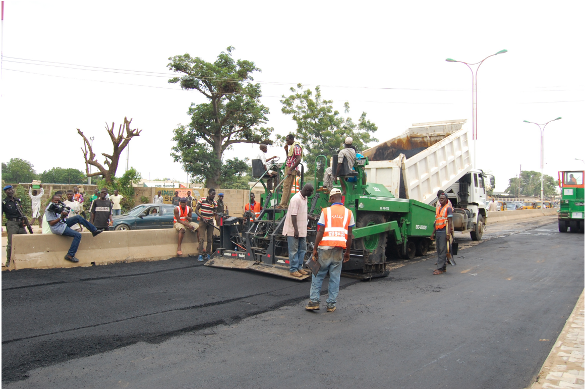
ASPHALT OVERLAY AT NEWLY COMPLETED CIVIC CENTER ROAD
