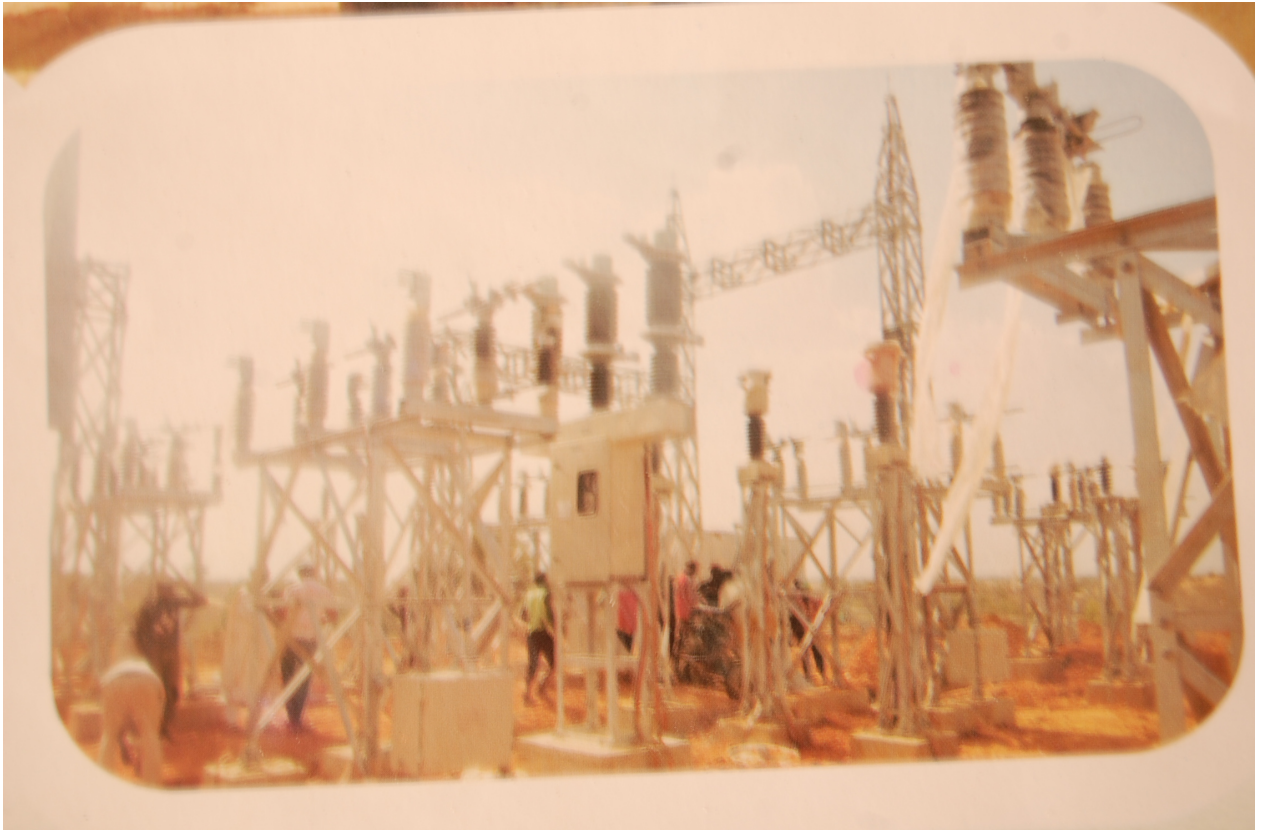
FIRST INDEPENDENT POWER PROJECT SITE AT TIGA.
