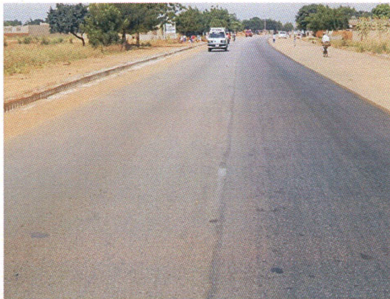
An almost completed 5-kilometre road in D/Kudu town, one of the 5-km road projects in all the 44 local government areas by the Kwankwaso Administration
